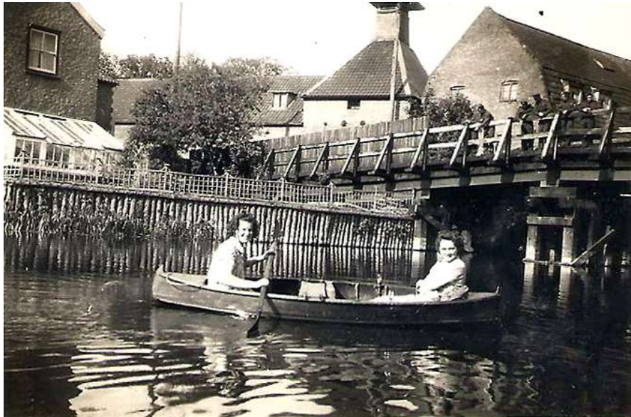
Brandon Bridge, 1943. Supplied by Pat Baldwin
