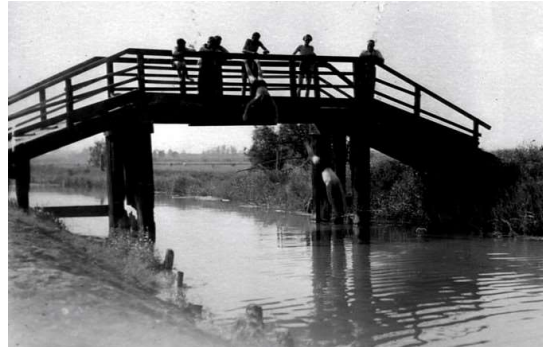
Diving off Burwell cock up bridge
