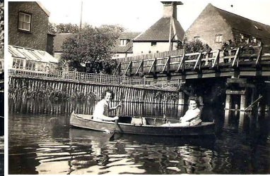
Mary Chapman and Eleanor Ridsdale, 1943 at Brandon Bridge, with temporary bridge
